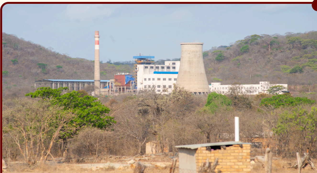
Brown Supply Chain: Coal powered electricity plant at Sabi Star lithium mine in Buhera where communities suffer energy poverty
