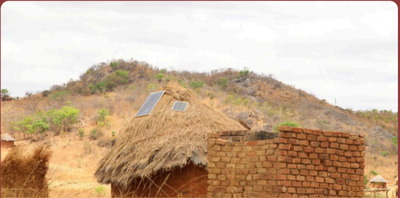
A traditional thatched homestead in Masvingo West Province, powered by the sun — where heritage meets clean energy and rural resilience shines.
