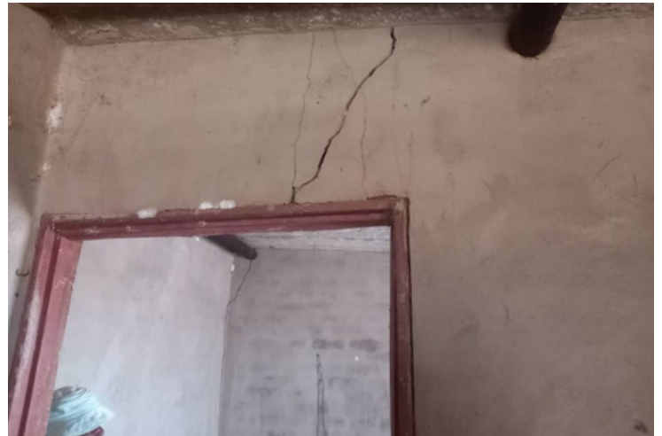
Blasting scars: A picture of a cracked house in Buhera
